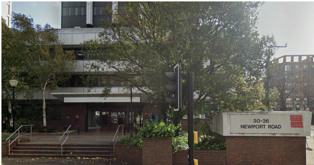
32 Newport Road in 2021. ©2022 Google
